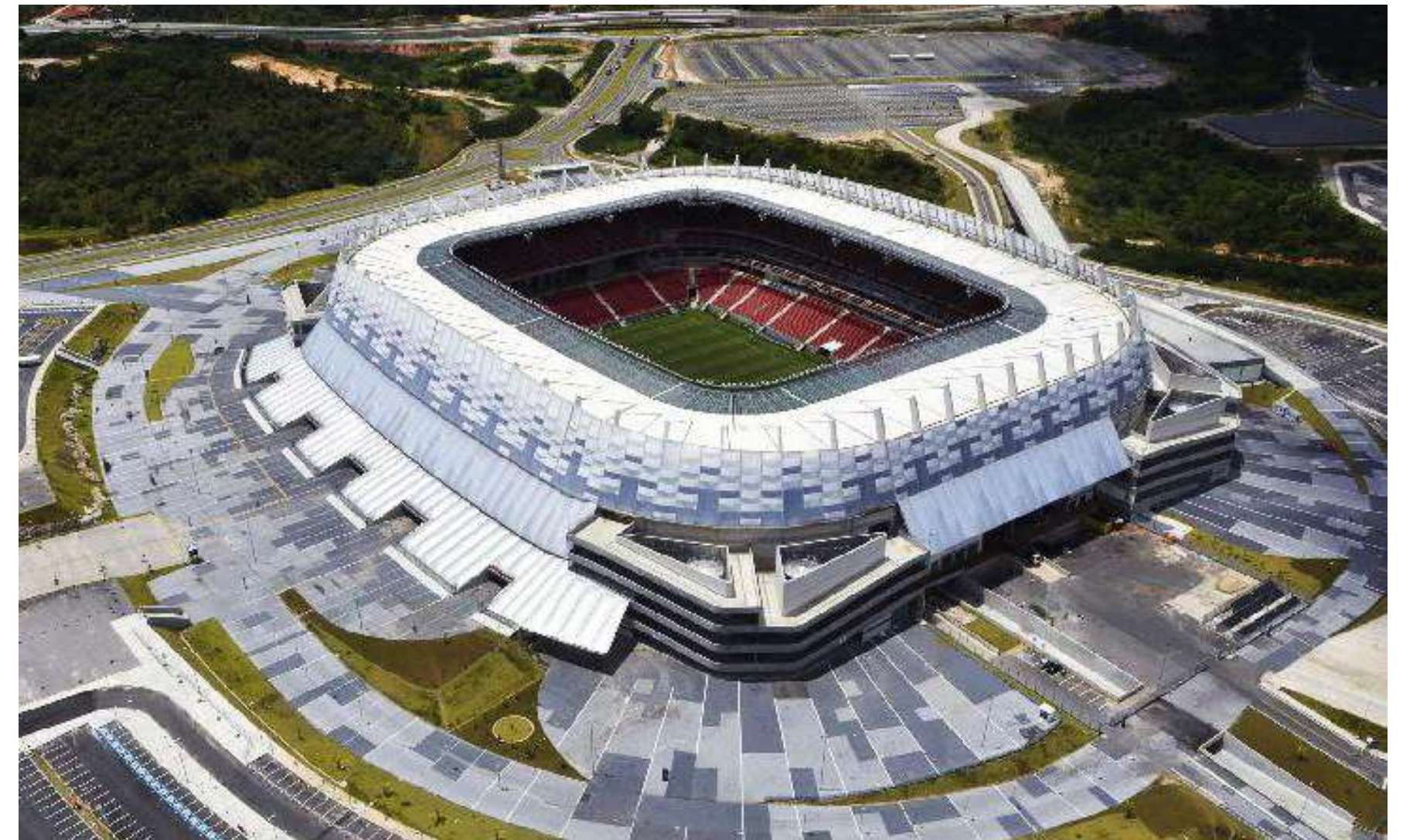
Arena Pernambuco Football Stadium | Brazil
